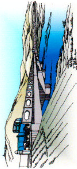
2. Reinforced concrete T-girder bridge with 4 spans, total length of 70 m
