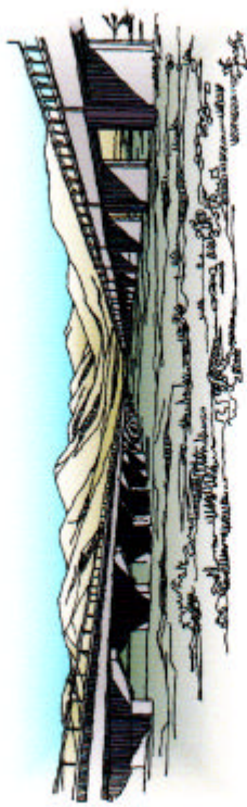
3. Additional Kherlen river bridge, prestressed concrete bridge with 8 spans, total length of 269 m
