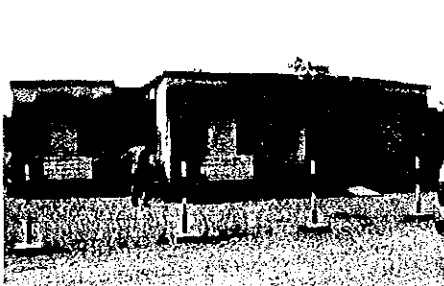
This is the SC constructed by DANIDA support. The right wing is residence of the health worker, and the left is for health care provision.
