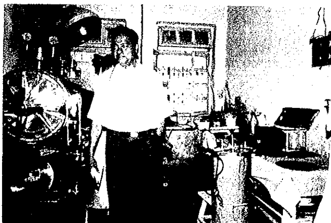
Sterilization unit for the operation theatre, Damoh District Hospital
