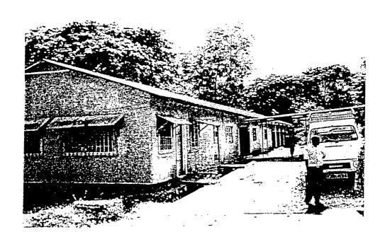
(BELOW) EXISTING WALKWAYS (SOME PORTIONS HAVE NO ROOF AND MAINLY COVERED BY OLD AND HAZARDOUS ASBESTOS SHEETS).
