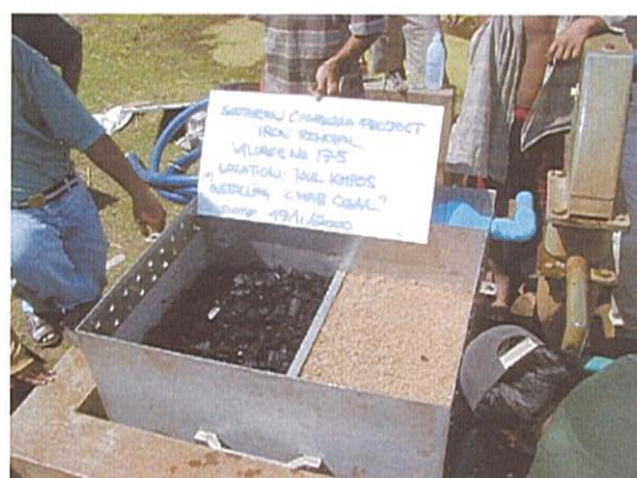
10. Filling charcoal into C chamber
