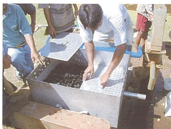
11. Cover C & D chamber by perforated plate
