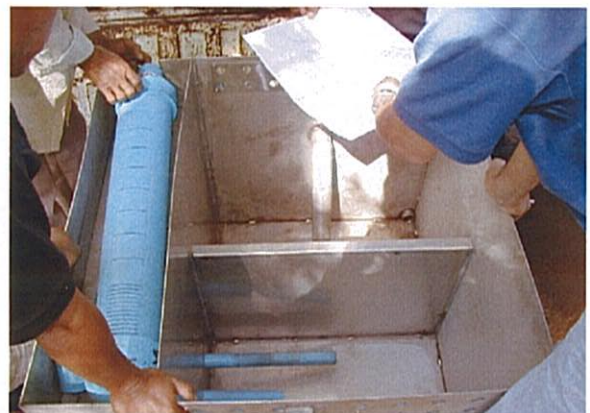
4. Setting inlet pipe into A chamber
