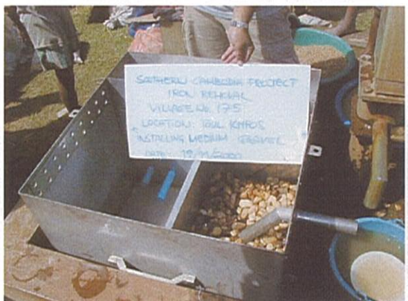
6. Filling medium gravel into D chamber
