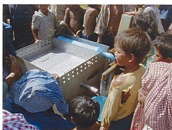
12. Connect flexible pipe to hand pump
