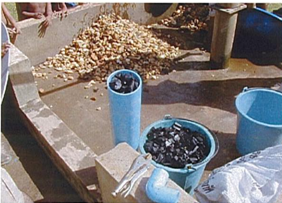
3. Filling charcoal into inlet pipe
