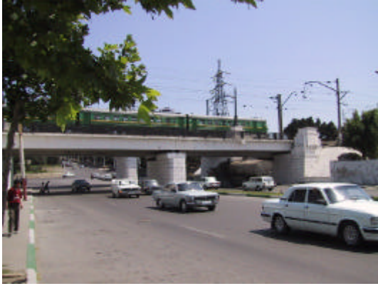
Grade Separation of Railway and Road
