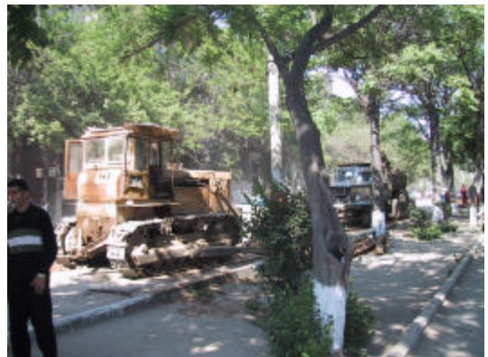
Road Repair Work
