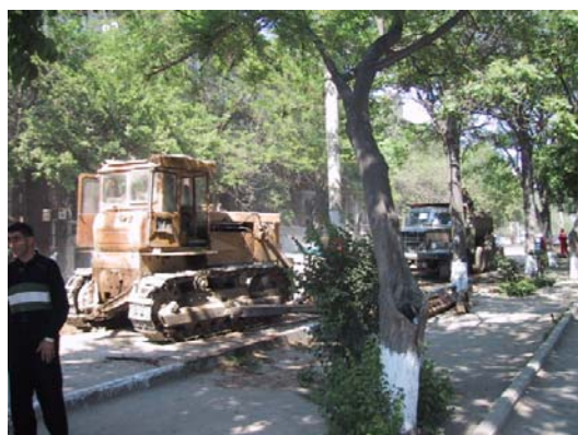
Road Repair Work
