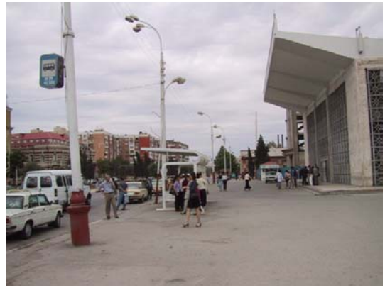
Frontage of Khatai Subway Station
