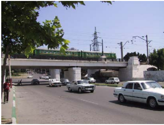
Grade Separation of Railway and Road
