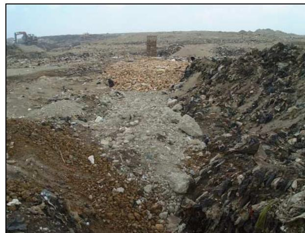
(Figure 10.6) Layers of the gravels applied to the leachate collection pipes
