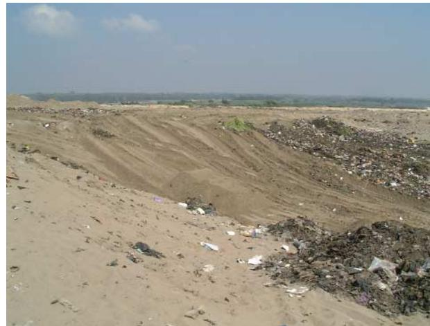
(Figure 9.4) Using the intermediate cover-soil in the working-phase 2
