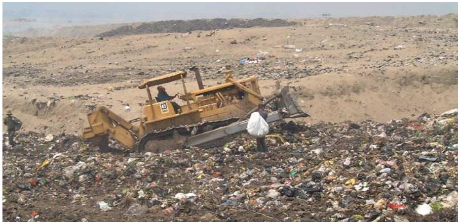
(Figure 8.8) Step 1: Compaction of the 1<sup>st</sup> layer of waste (forming a slope of 1:4)
