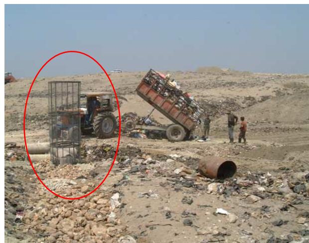
(Figure 9.6) 1<sup>st</sup> part of the gas removable collection pipe (steel casing and perforated concrete pipe)
