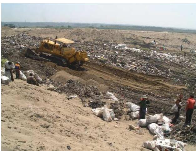
(Figure 8.10) Bulldozer is pushing the sand in order to form a 10 cm layer of intermediate cover-soil as well as good compaction of the waste
