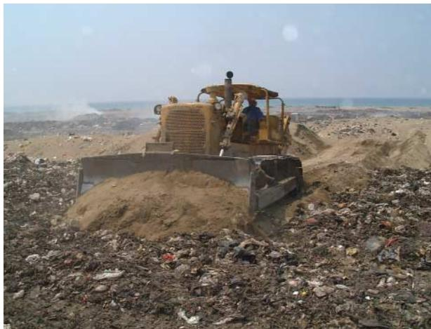
(Figure 8.5) Covering the cell of the compacted waste of week 7
