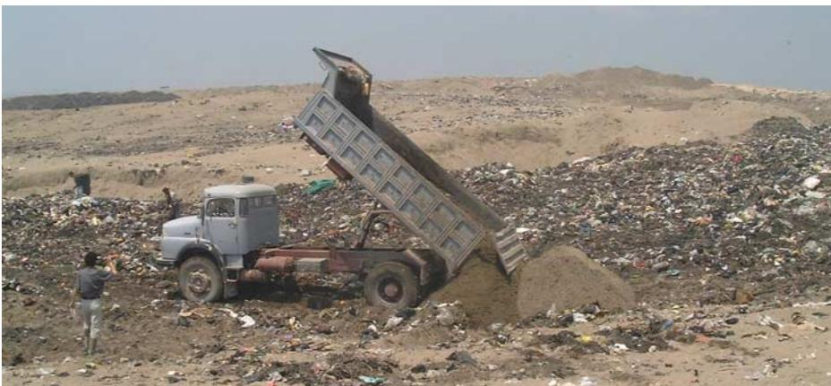
(Figure 8.9) Step 2: Discharging some sand by the dump truck
