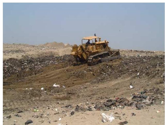
(Figure 8.11) The bulldozer, in working-phase 2, is spreading the intermediate cover-soil
