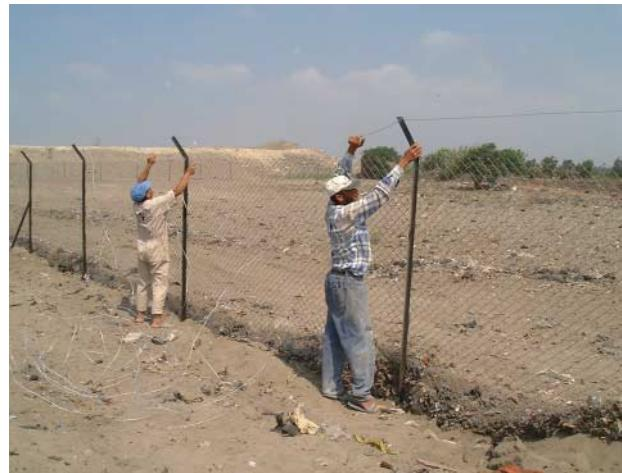
(Figure 8.13) Installation of the upper steel wires of the fence
