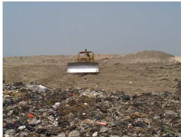
(Figure 8.6) Compacting the cover-soil
