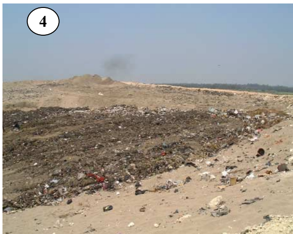
<Landfill Operation (Cell Method) with Waste Compaction and Cover Soil>
