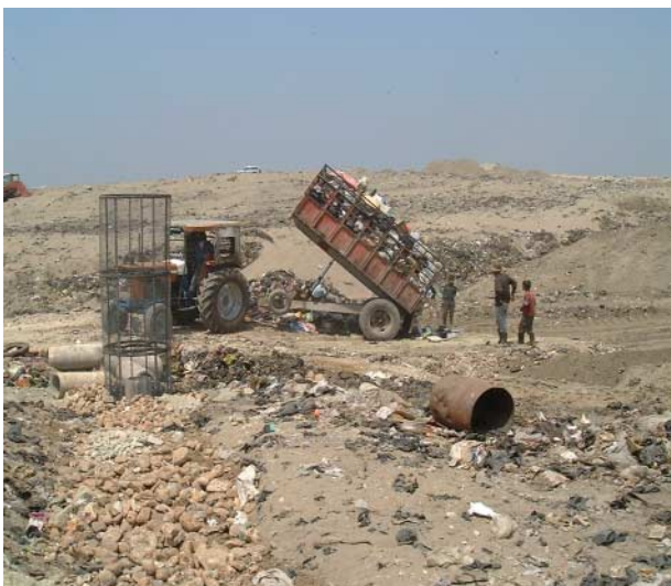
Gas Removal Pipe
