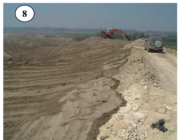
<Rearrangement of Existing Accumulated Waste as a Core of Embankment>
