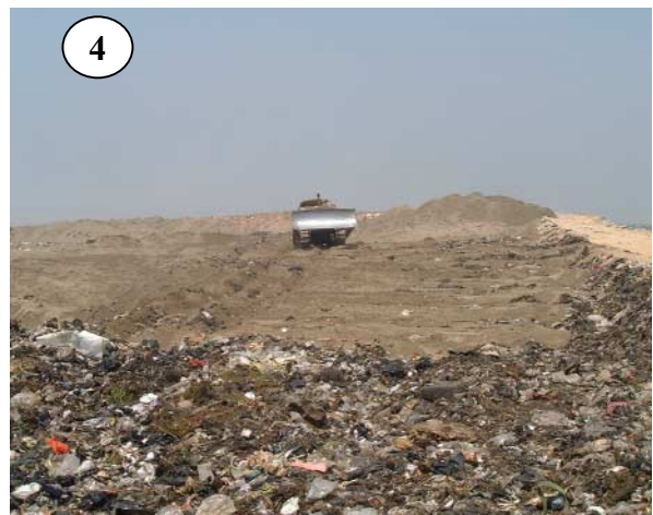
<Landfill Operation (Cell Method) with Waste Compaction and Cover Soil>
