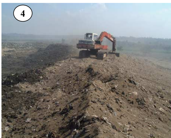
<Rearrangement of Existing Accumulated Waste as a Core of Embankment>
