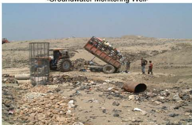
<Gas Removal Pipe>
