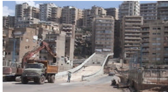
On-going Grade Separation Project
