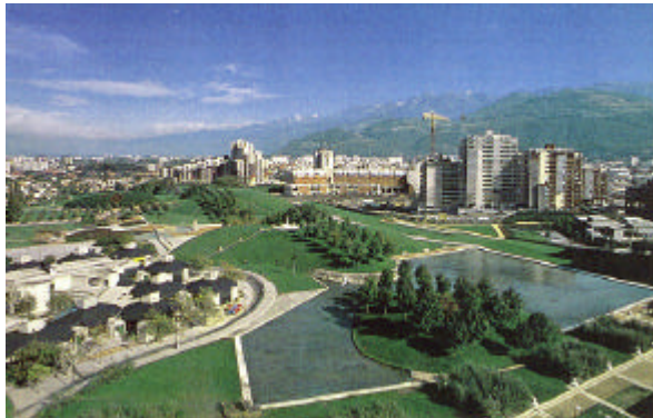
Image of Old and New Development Areas [La Villeneuve de Grenoble – France]
