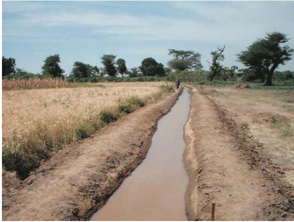
Irrigation Canal Completed
