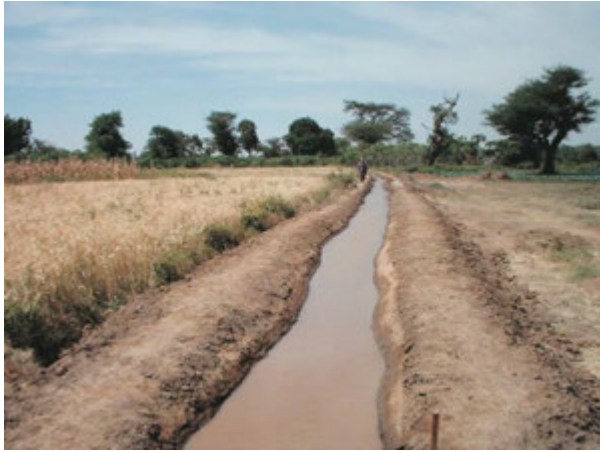
Irrigation Canal Completed
