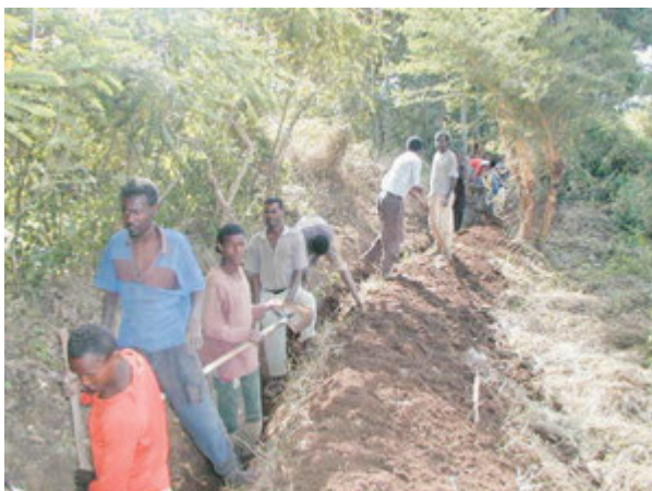
Participatory Canal Construction
