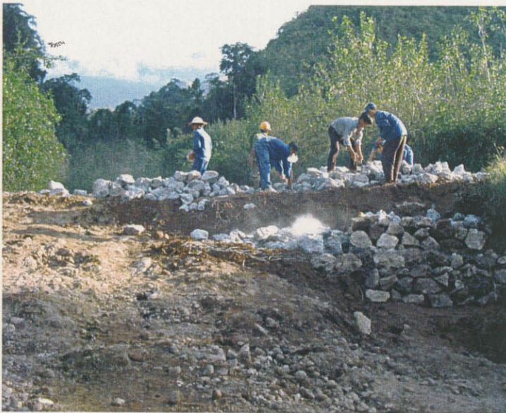
Reinforcement of road cross part of the river (Work of TERRAPRODEX)
