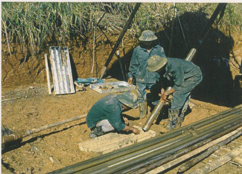
Extraction work of core
