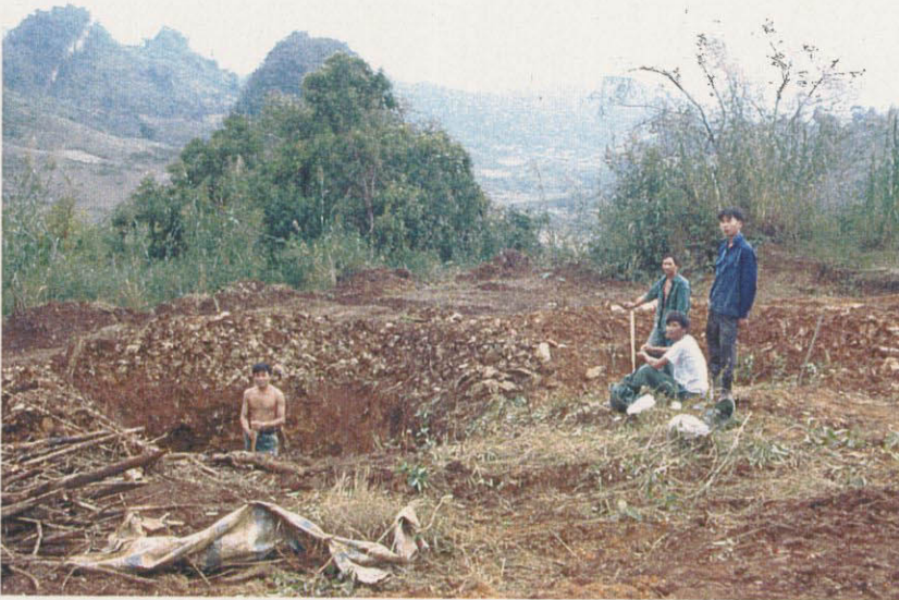
Construction of pool for drilling mud
