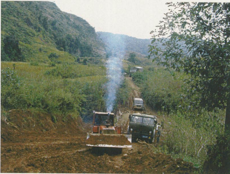
Carry-in situation of drill equipments by help of bulldozer
