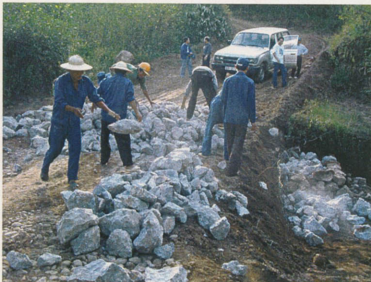
Almost construction work was done by human power (Work of TERRAPRODEX)
