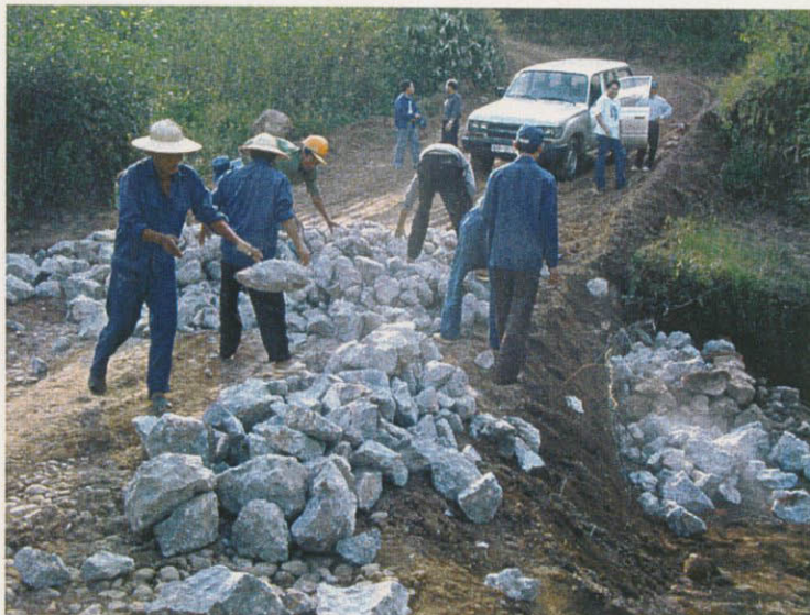
Almost construction work was done by human power (Work of TERRAPRODEX)
