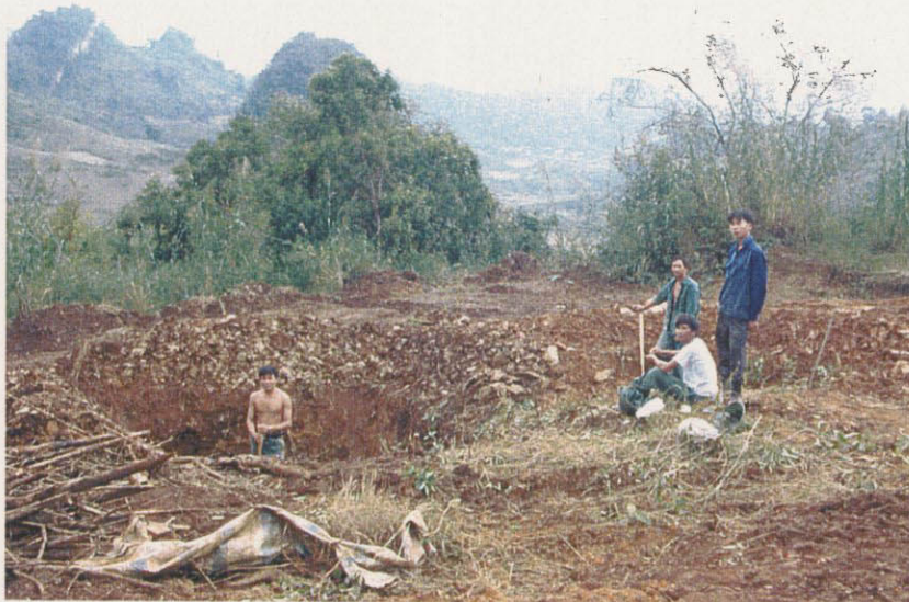
Construction of pool for drilling mud
