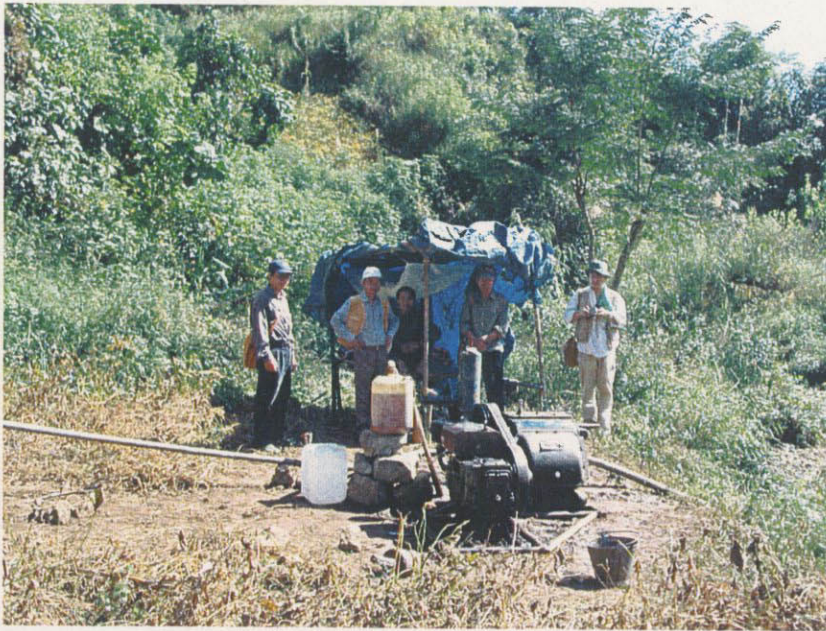
Water pump (Dong Pao river site)
