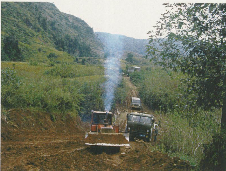
Carry-in situation of drill equipments by help of bulldozer
