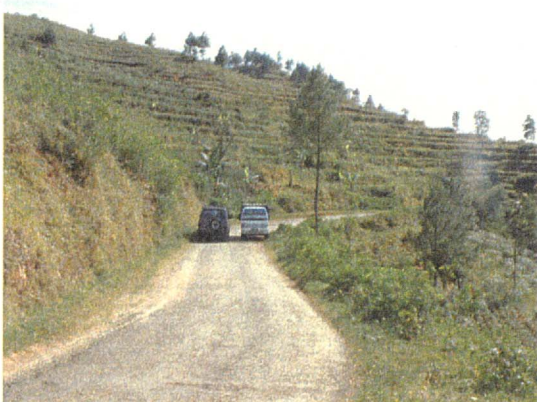
(3) Road in the Southern Part of the Survey Area
