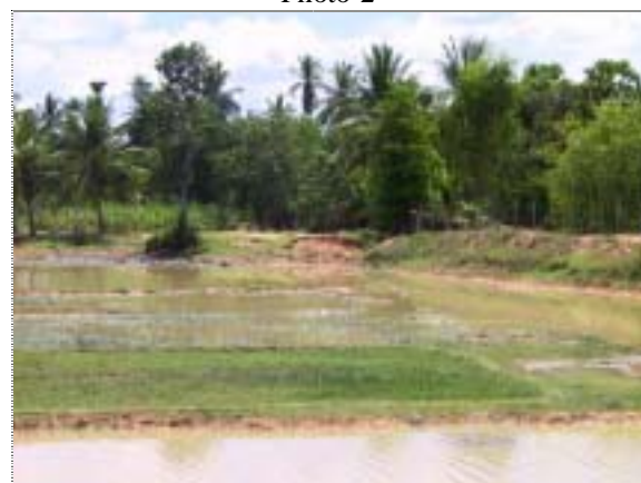
Dike was flushed by the stored water
