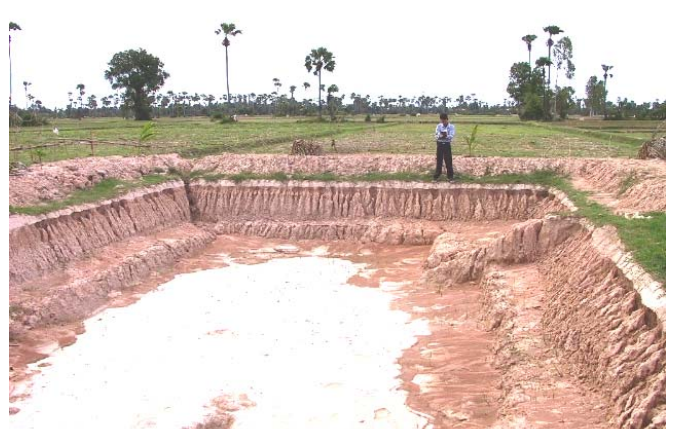
PDP Area Under Construction of Pond at Trapeang Snao Village
