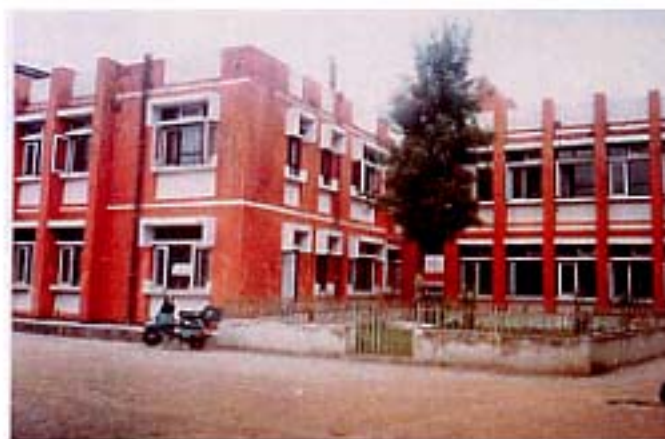
The major structure of Teku Hospital: Two story masonry building
