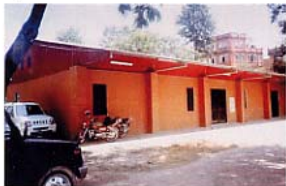
Earthquake resistant one story building of Bhaktapur Hospital
