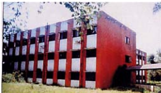
Main building of Bhaktapur Hospital: Three story masonry building
