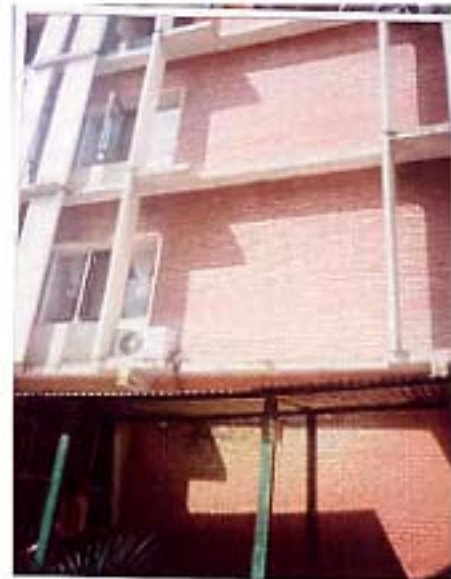
Four story masonry Building: Needs some improvement
