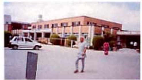
Two story frame building of Teaching Hospital
