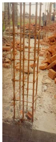
Foundation base reinforcement
