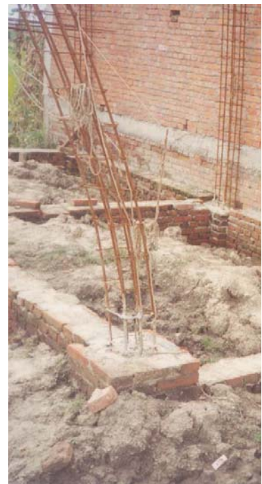
Erection of column bars
