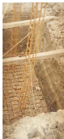
Foundation base reinforcement
