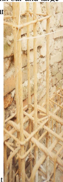
Improper anchorage of beam bars
