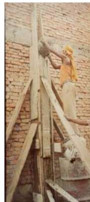
Concreting work in column
