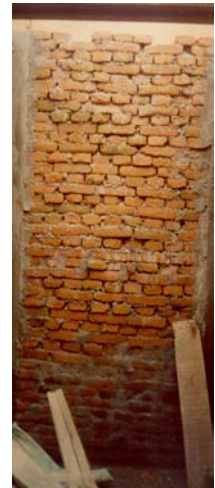
Poor quality Brick work
