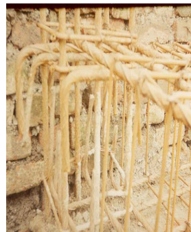
Improper anchorage of beam bars
