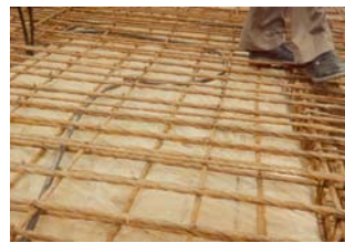
Slab Reinforcement
