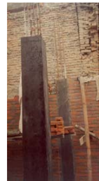
Column Reinforcement and Concreting work
