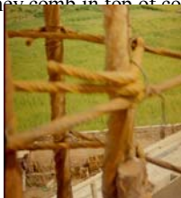
Proper tie hooks
