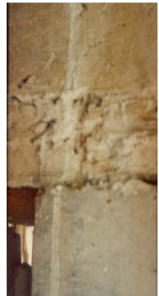
Beam column joint with honey combing
