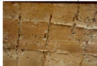
Beam column joint with honey combing
