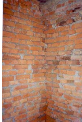
Three story masonry building under construction, Ground floor in mud mortar and remaining floors in cement mortar
