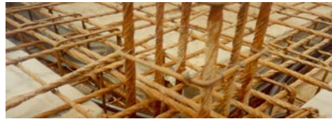
Column tie hooks bent at 90°
