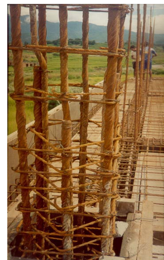
Column bars splices in staggered position
