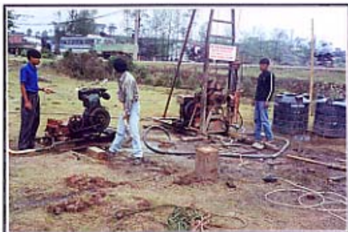
Core Drilling at Thini Madhyapur (BH # 4)
