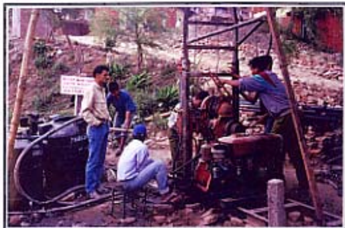
Core Drilling at Singh Durbar, Kathmandu (BH # 2)
