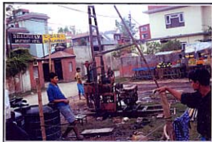
Core Drilling at Jawalaket, Lalpur (BH # 3)
