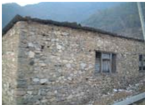
Photo 1.8.1 Stone with mud mortar (ST)
