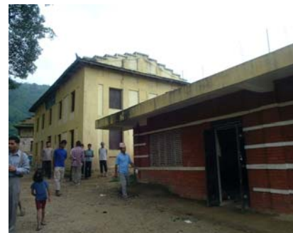
Photo 6.1.17 Retrofit to School
