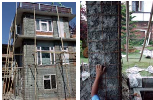
Photos 6.1.15 and 16 Jacket Reinforcement
