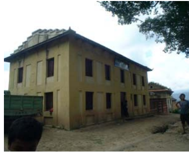
Photo 6.1.12 Retrofit to school
