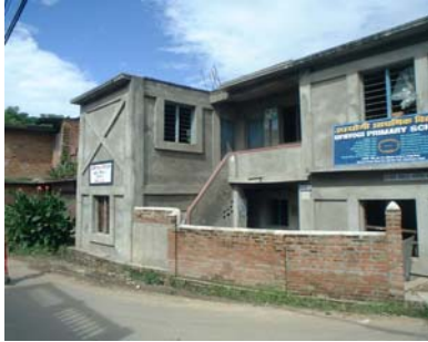
Photo 6.1.11 Retrofit to school
