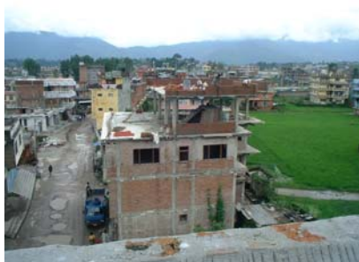
Photo 6.1.1 RC frame with masonry
