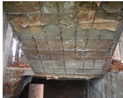
Photo 6.1.8 RC Structure (lapping length shortage)
