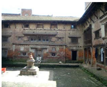
Photo 6.1.10 AD structure with courtyard
