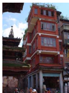
Photo 6.1.2 Cantilever Structure
