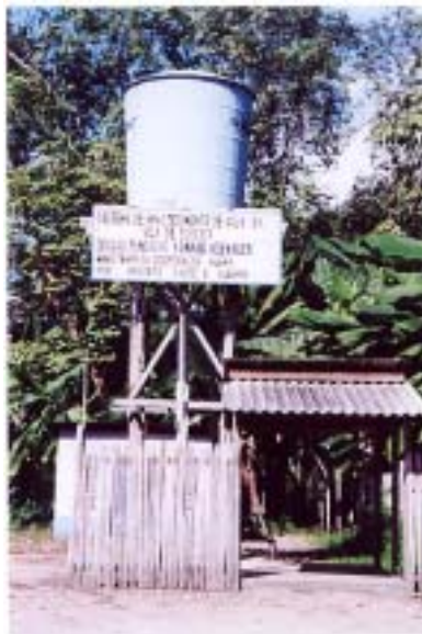
Rural Water Supply Facility
