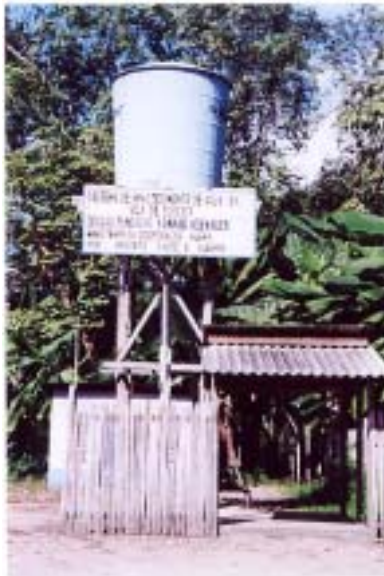
Rural Water Supply Facility
