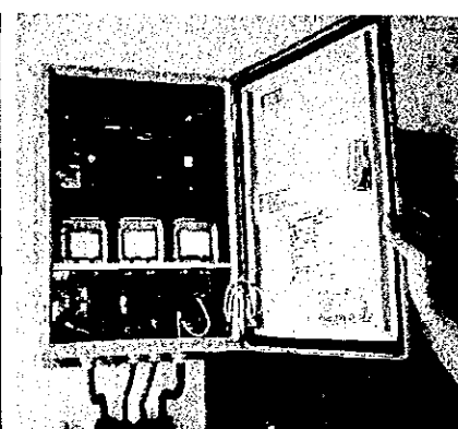
Inverter of Solar generating System
