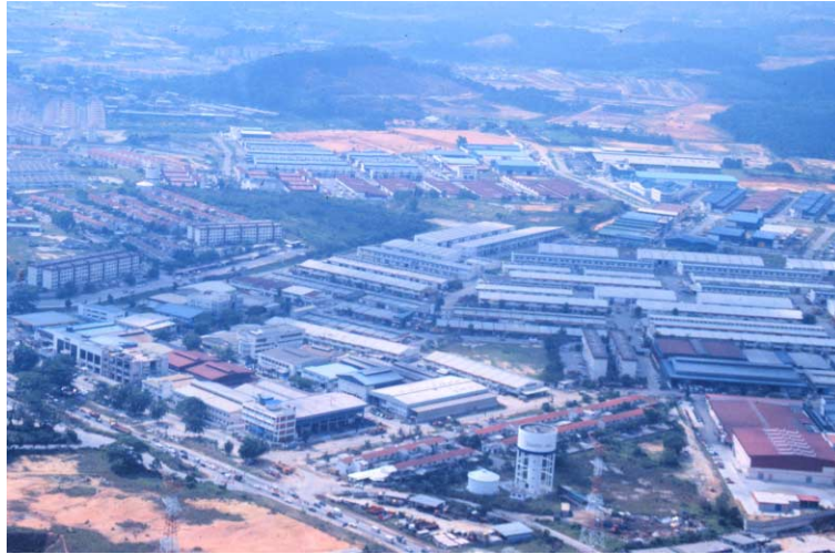
Photograph E.4.1 Industrial Estates in Balakong, Hulu Langat
