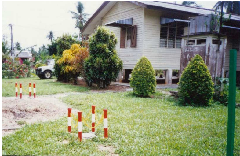
Photograph H.4.1 Finished Benchmark Station (BM1: Left) and Datum Point (DP1: Right)
