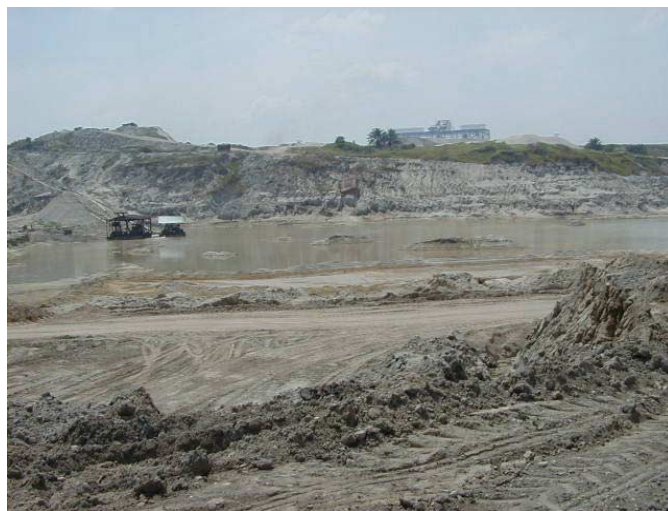
Photograph E.4.5 Active Mine near Megasteel, Dengkil (2)
