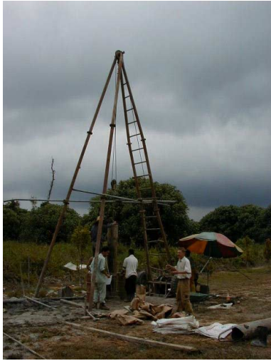
Drilling of Monitoring Well along the ELITE Highway 13/2/2001
