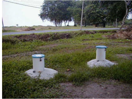
One of New Monitoring Wells 13/9/2001
