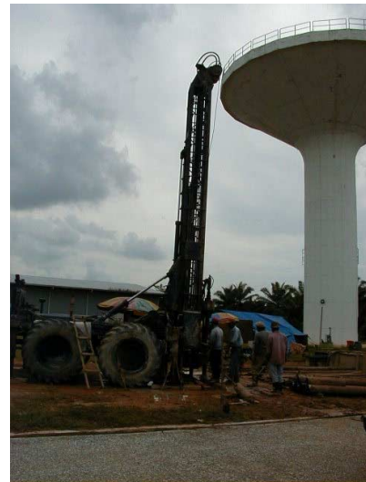
Drilling of Monitoring Well at Kajibumi WF2 23/10/2000
