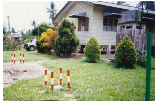
Establishment of Land Subsidence Monitoring Benchmarks 7/8/2000
