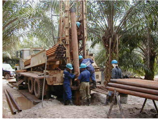
Drilling of Monitoring Well at Kanchong Darat 13/2/2001
