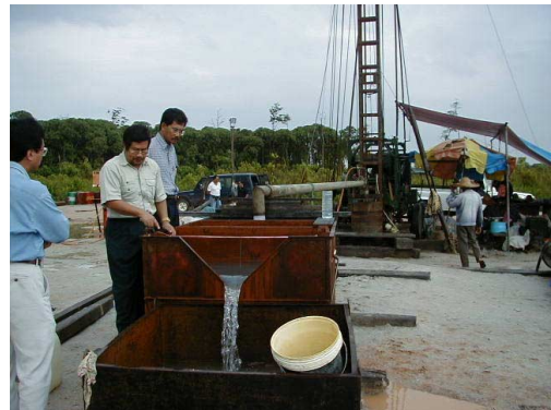
Pumping Test at Kanchong Darat 13/2/2001
