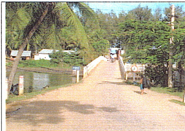
Picture 1: On bridge center line
