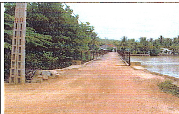
Picture 1: On bridge center line
