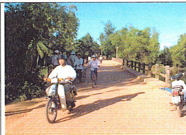
Picture 1: On bridge center line
