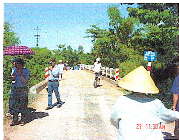
axis direction from the right bank
