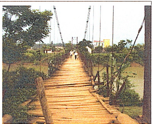
axis direction from the right bank
