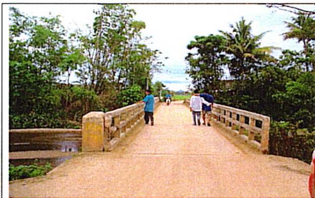
Picture 1: On bridge center line
