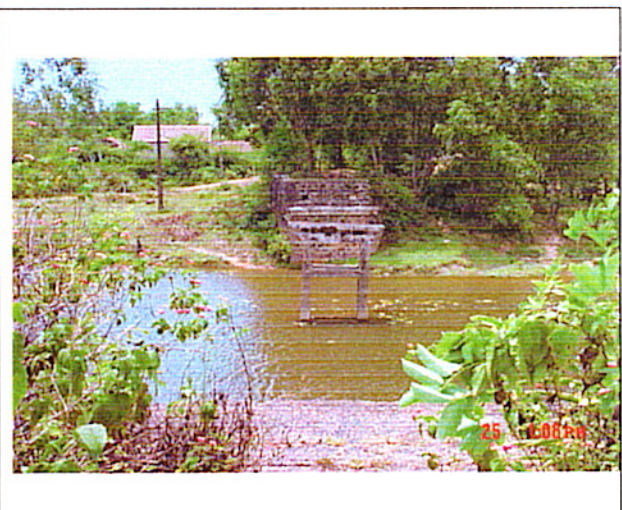
Picture 2: The former bridge on the bridge alignment from left bank
