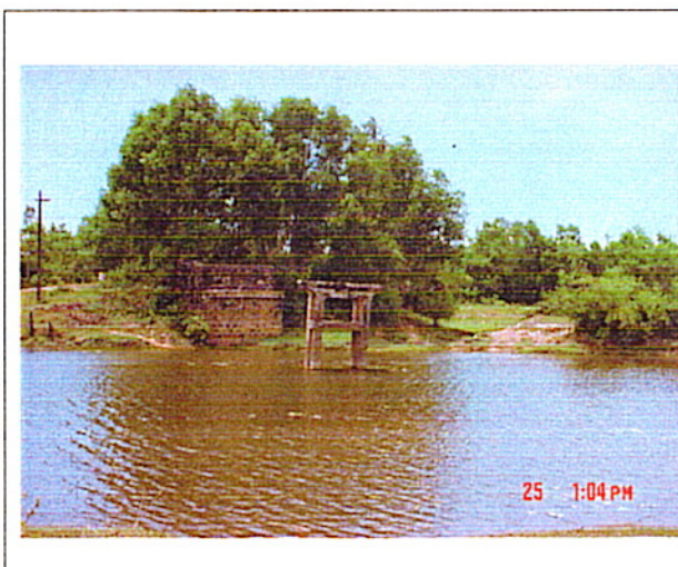
Picture 1: The former bridge from the left bank
