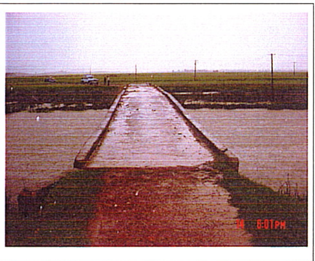
Picture 2: The existing bridge from left bank
