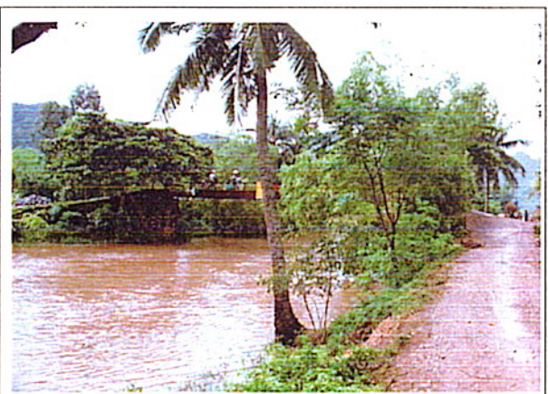
Picture 2: Approach road on right bank, down-stream, and 2.0m wide only
