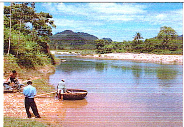
Picture 2: From down stream. On right bank abutment of former bridge (washed Away) is seen.
