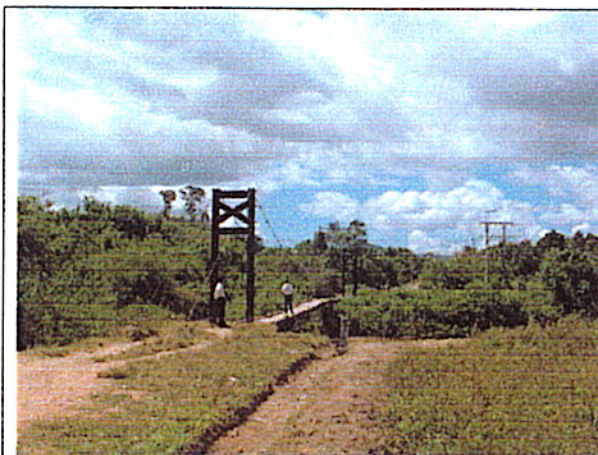
Picture 1: On the alignment of proposed bridge (after demolition of existing one)
