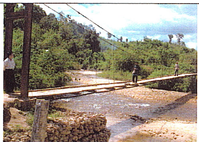
Picture 2: From upstream
