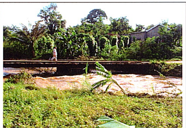
Picture 2: Existing Bridge
