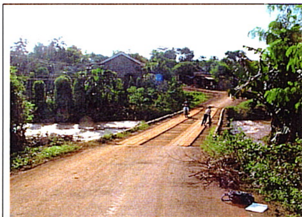
Picture 1: Existing Bridge
