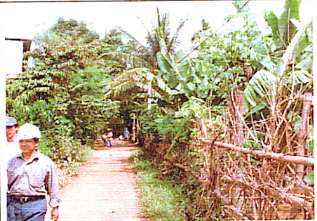
Picture 2: Access road on right bank is narrow, 3m only. Several houses on downstream (right side of photo) shall be removed.
