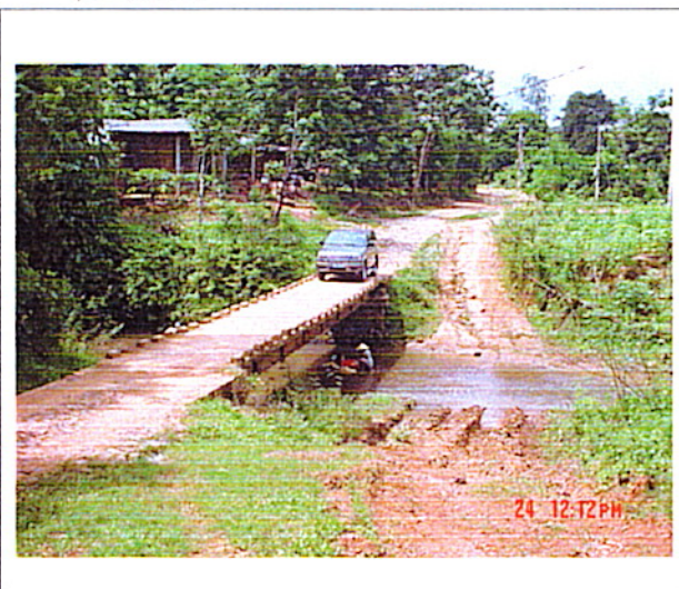
Picture 1: The existing bridge from right bank
