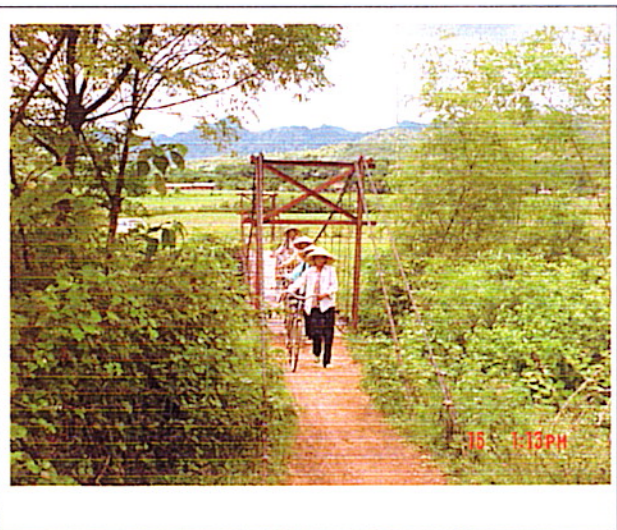
Picture 2: The existing bridge from left bank
