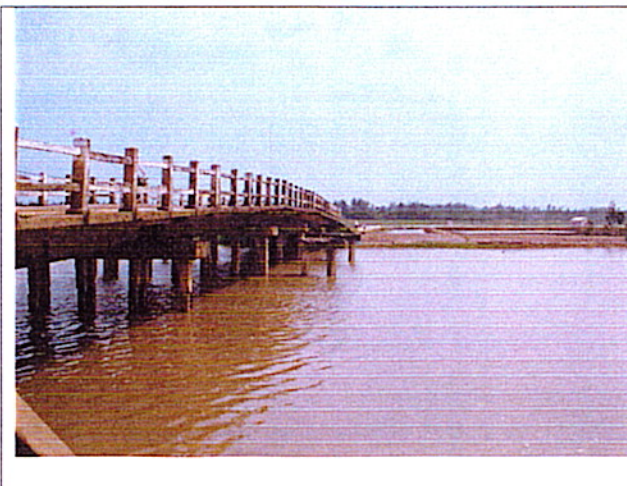
Picture 1: On proposed bridge alignment from right bank, 2 protection pile groups to be removed.
