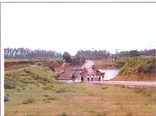
Picture 1: From left bank. At left end of photo The proposed alignment of bridge will be allocated.
