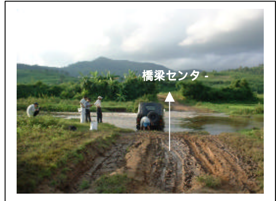
Photo-6 NO.62 Ngoc Reo Bridge (Kon Tum Prov.)
