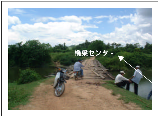
Photo-7 NO.72 Song Sau Bridge (Quang Ngai Prov.)
