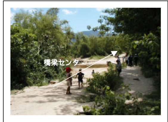
Photo-8 NO.82 Da Lac Bridge (Phu Yen Prov.)
