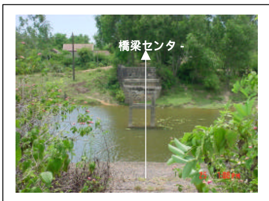
Photo-3 NO.20 Ben Da Bridge (Quang Binh Prov.)
