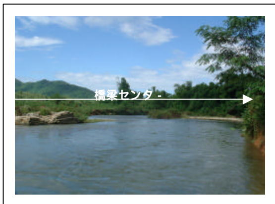
Photo-3 NO.27 Hoi Phuoc Bridge (Da Nang City)
