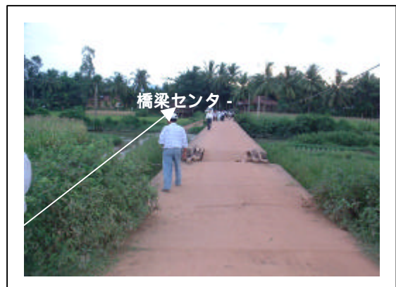
Photo-6 NO.67 Xa Cai Bridge (Quang Ngai Prov.)
