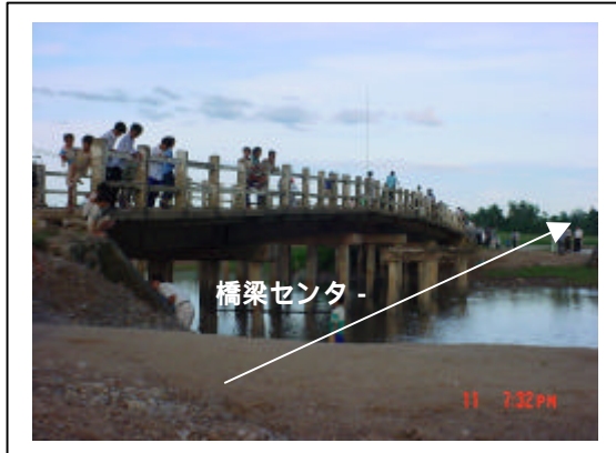
Photo-1 NO.6 Quynh Bang Bridge (Nghe An Prov.)
