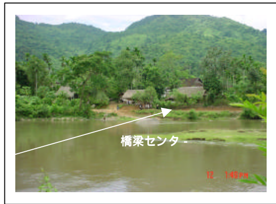
Photo-2 NO.9 Ban Khoang Bridge (Nghe An Prov.)
