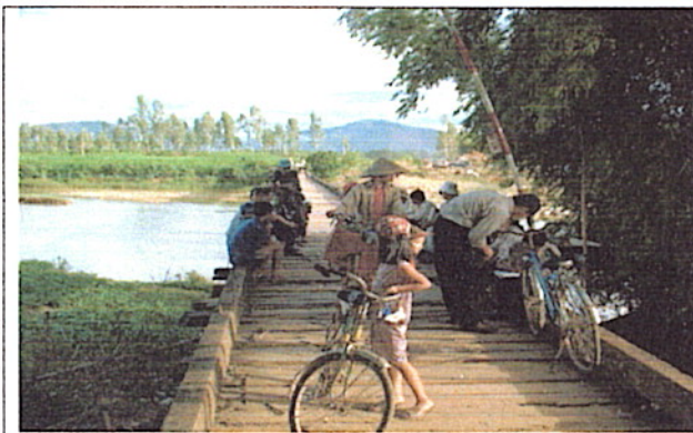
Picture 1: On bridge center line
