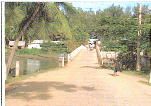
Picture 1: On bridge center line
