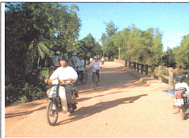
Picture 1: On bridge center line
