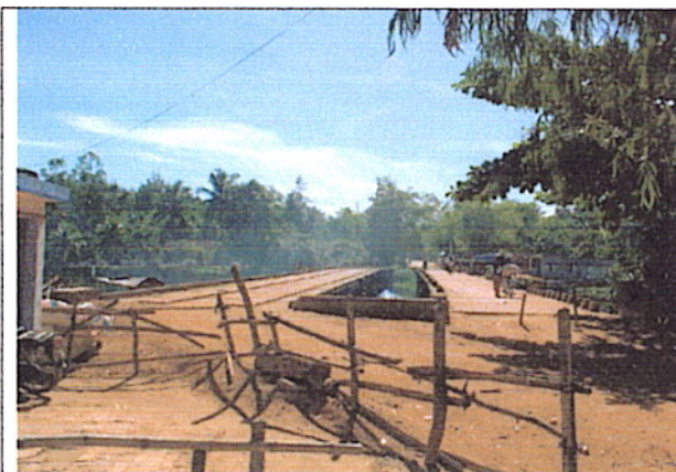
Left: New temporary with steel girder, Right: Old concrete
