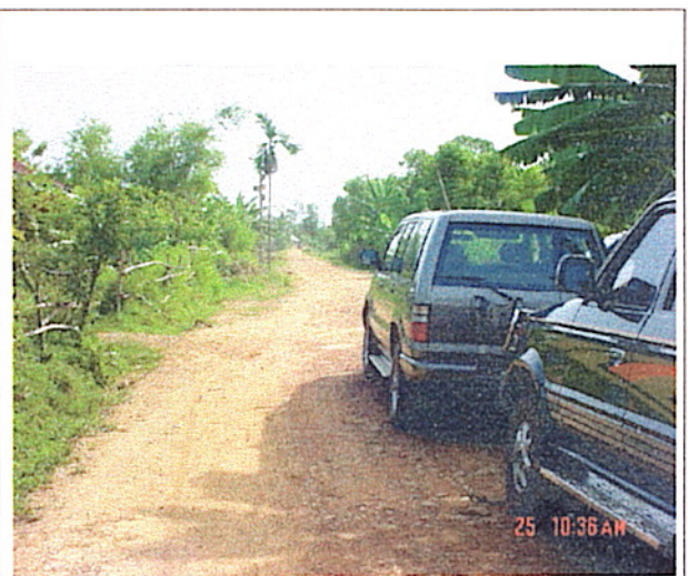
left-bank approach road
