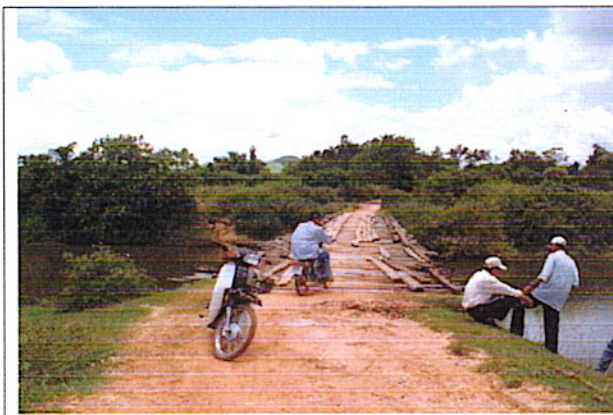
Picture 1: On bridge center line from left bank
