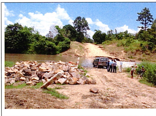
Picture 1: On bridge center line
