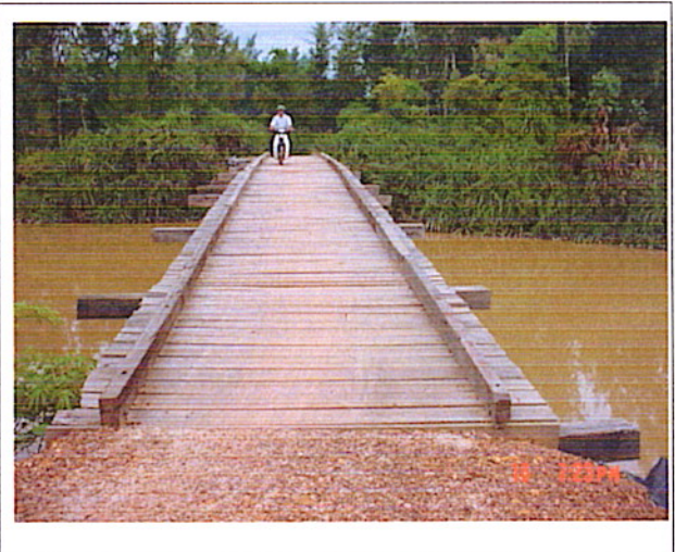
Picture 2: The existing bridge from the left bank
